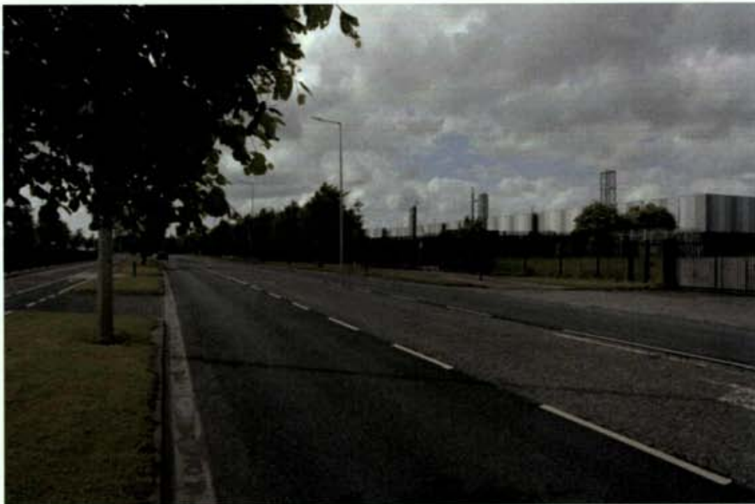
Figure 11.3 View along Cruiserath Road to the south of the overall development lands illustrating the completed Data Centre Building A and southern perimeter landscaping
