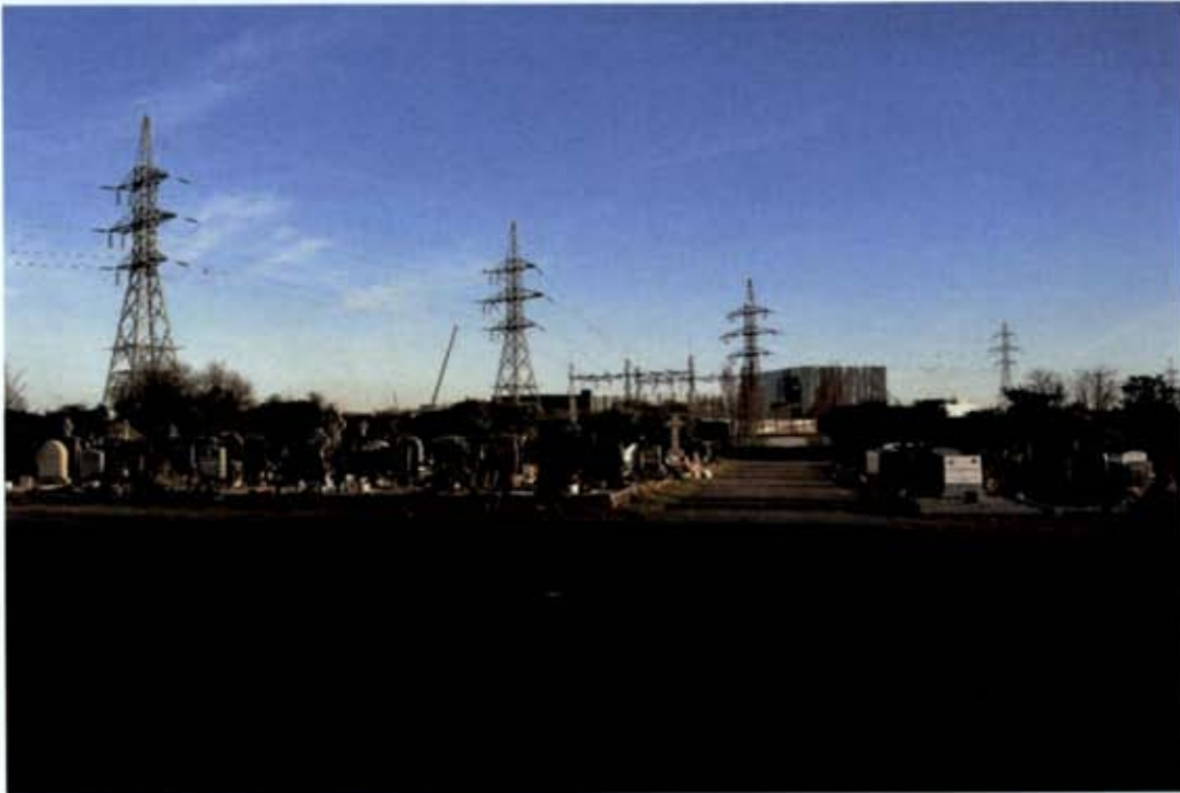
Figure 11.8 View from entrance gate to Mulhuddart Cemetery at Church Road looking east and showing the 110kV pylons, ESB substation and Alexion beyond the cemetery in the foreground.
